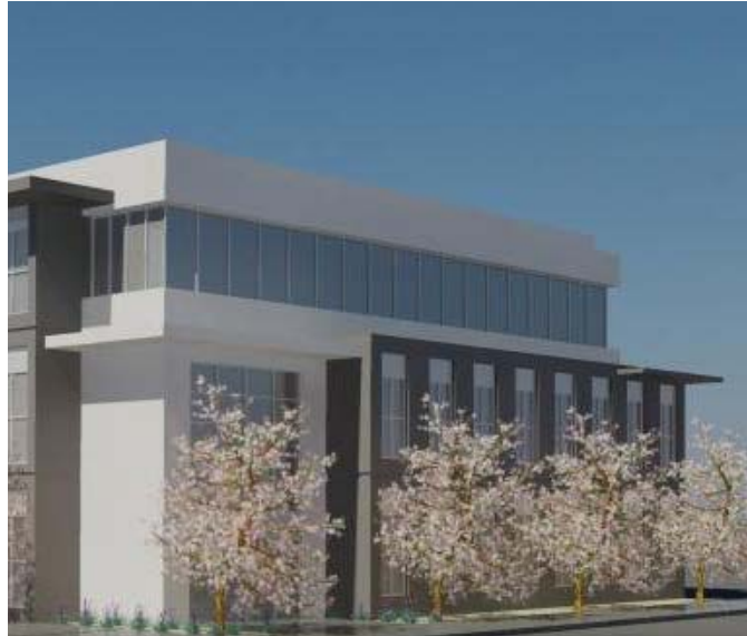
Clinic, South face, from the Intermodal Hub
